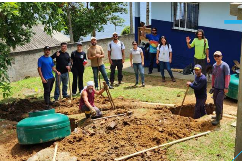
Joint effort to install an ecological effluent treatment system in Eufrasina
