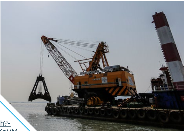
Maintenance dredging in the access channel
